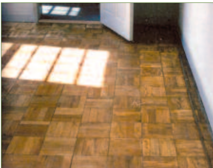
The before, showing carpet glue, tack strip, scratches and plenty of abuse.
