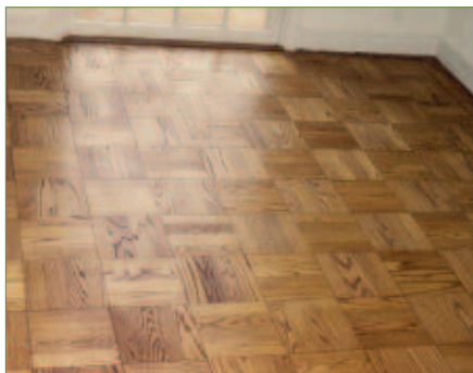
The finished floor; the scratches, uneven bevels, gouges, and some uneven areas are not prominent features when viewed from a standing position. The result: a very satisfied customer.
