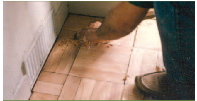
The loose slats along the left wall had to be reinstalled for sanding.
