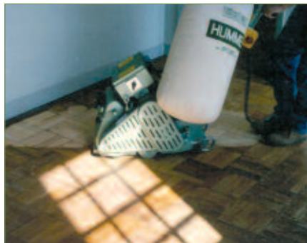
The beginning: sanding on an angle to flatten the flooring.
