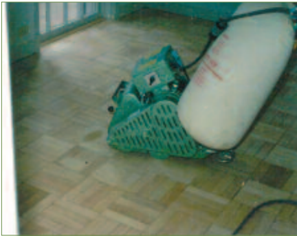
This photos shows sanding around the gouge after the second application of filler.
